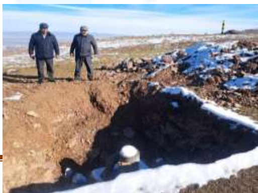
1-rasm. Bosh referens geodezik punktni Samarqand shahri Chuponota tepaligida qurish jarayoni
