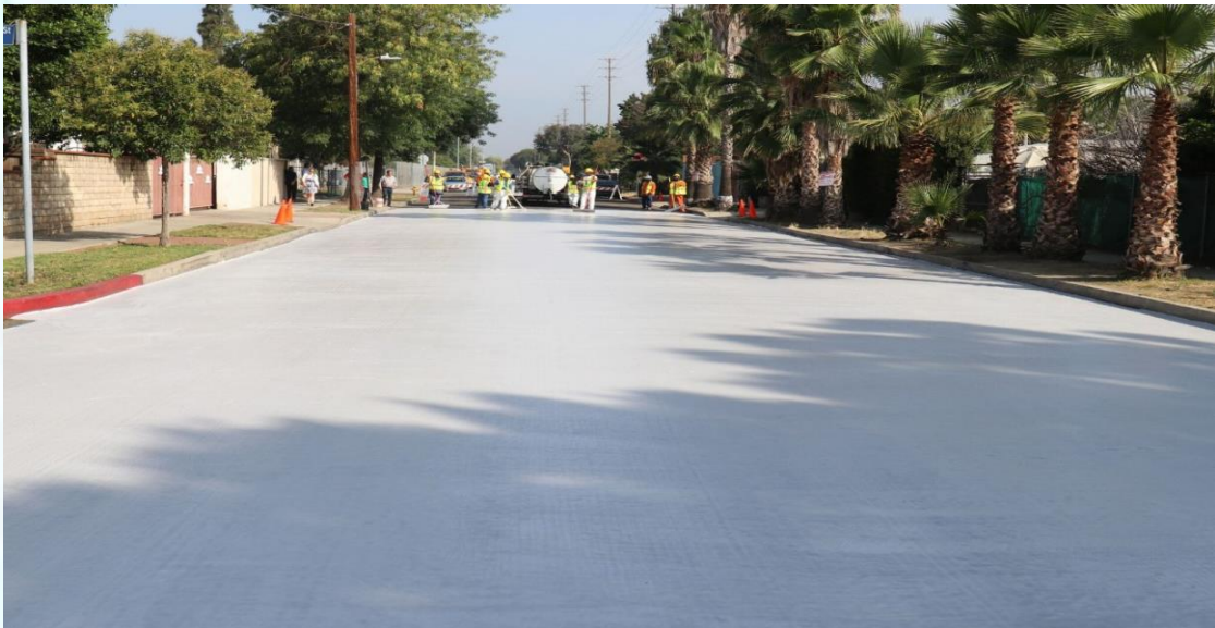
2-rasm. Porloq asfalt (cool pavement)
